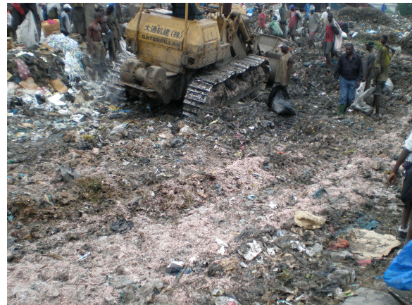
Fig 6.7 Bulldozer compacting after sorting
