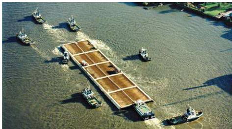
**Figure 3.2:** Tug boats manoeuvring an immersed tunnel element. (ITA 1999)
