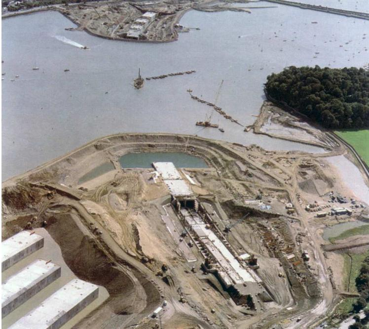
**Figure 3.1:** The Conwy tunnel in Wales during construction (1988). The connection tunnels are fully constructed, and plugged with bulkheads. The completed immersed tunnel elements in the dry dock can be seen in the lower left corner. (DGF 2005, p140)
