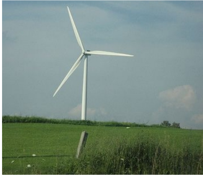
Fig. 1.9: GE 1.5 XLE wind turbine [32].
