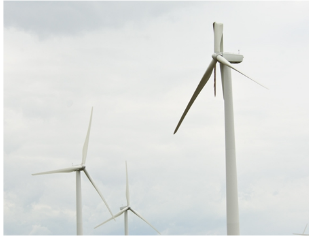
Fig. 1.2: Wind turbine with a failed blade [10]. The wind turbine is located near Wilton, North Dakota, USA.
