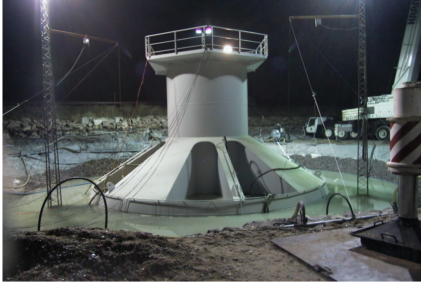
Figure 1.2. Installed bucket foundation at Frederikshavn Havn. [Larsen, 2008]
