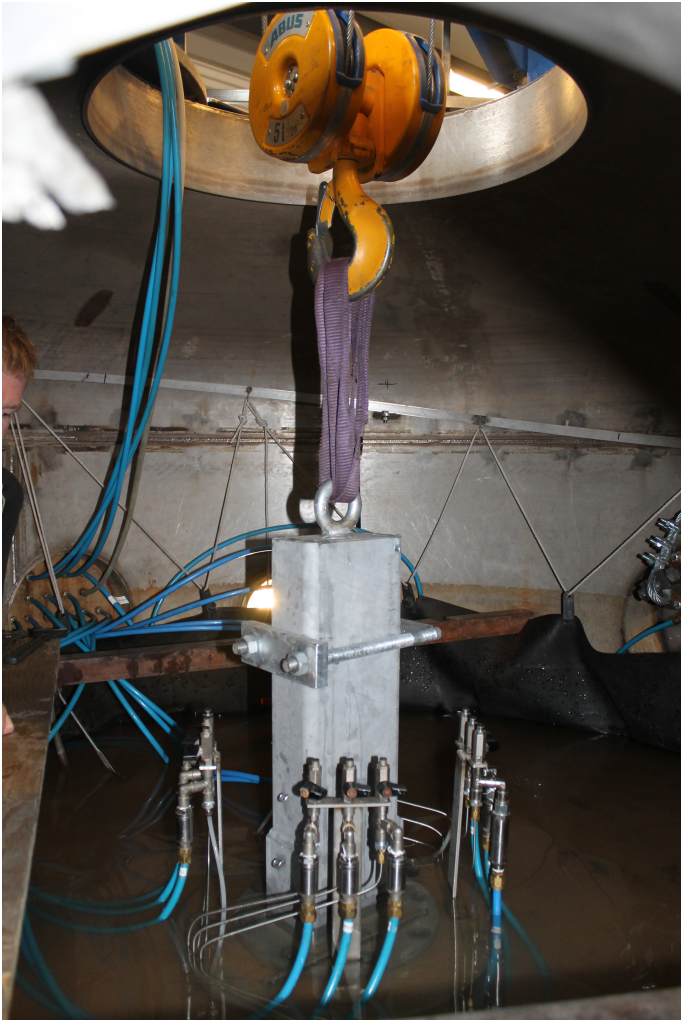
Figure H.9. Mounting the tower on the installed bucket.
