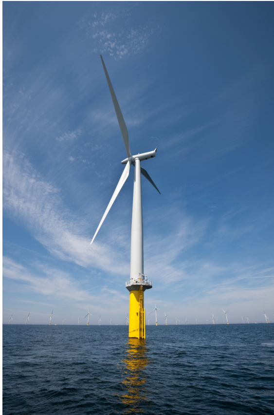
Figure 1.1. The Siemens 3.6 MW wind turbine used at Horns Rev 2 in Denmark. [DONG Energy, 2009]
