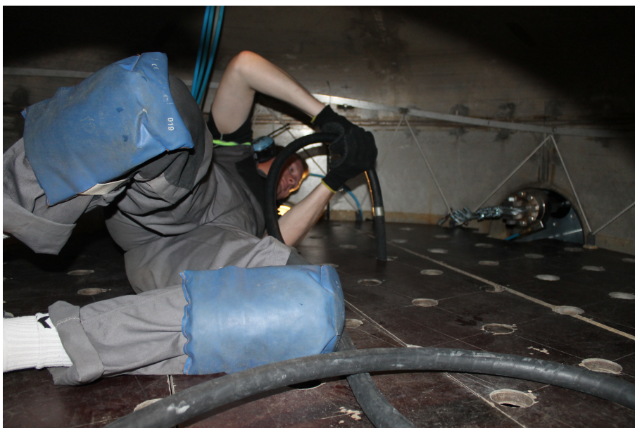
Figure H.3. Vibrating the sand.
