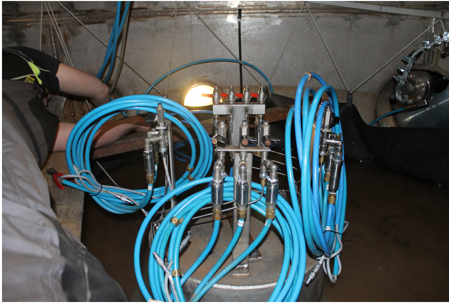
Figure H.7. The bucket placed on the aluminum plate, cables ready to be lead out of the tank.
