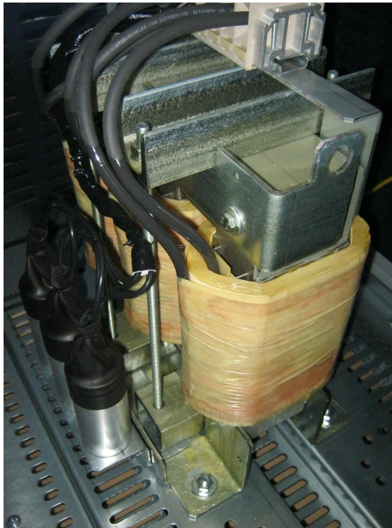
Fig. 2.7. 115 (A) three-phase LC-filter used between the VLT and the transformers
