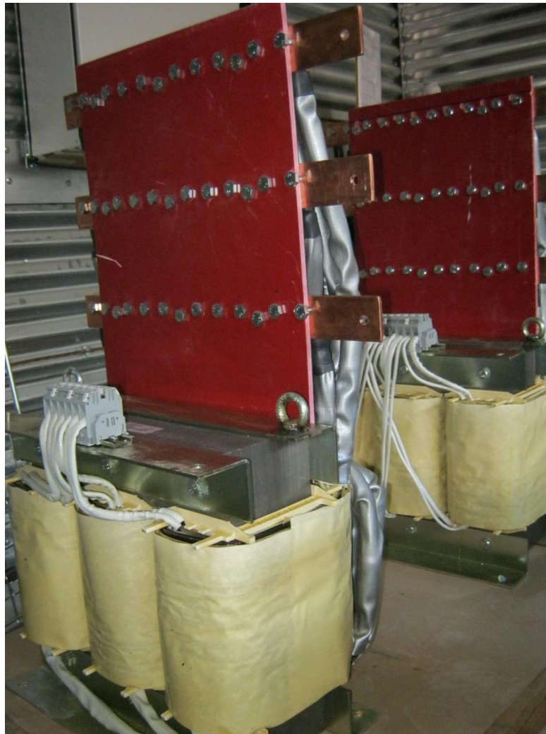
Fig. 2.10. Picture of the transformers used for power supply the 3000 (A) DC-link
