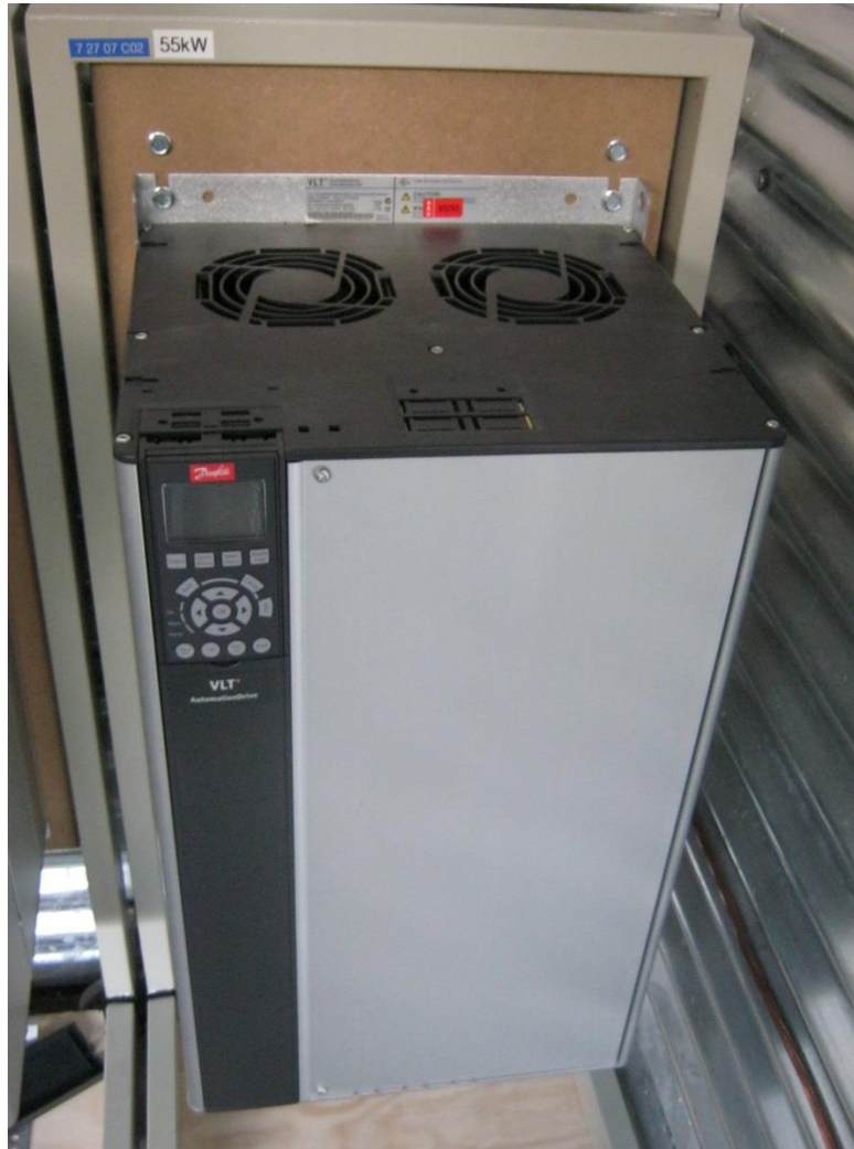
Fig. 2.6. Picture of the Danfoss VLT frequency converter used for power supply
