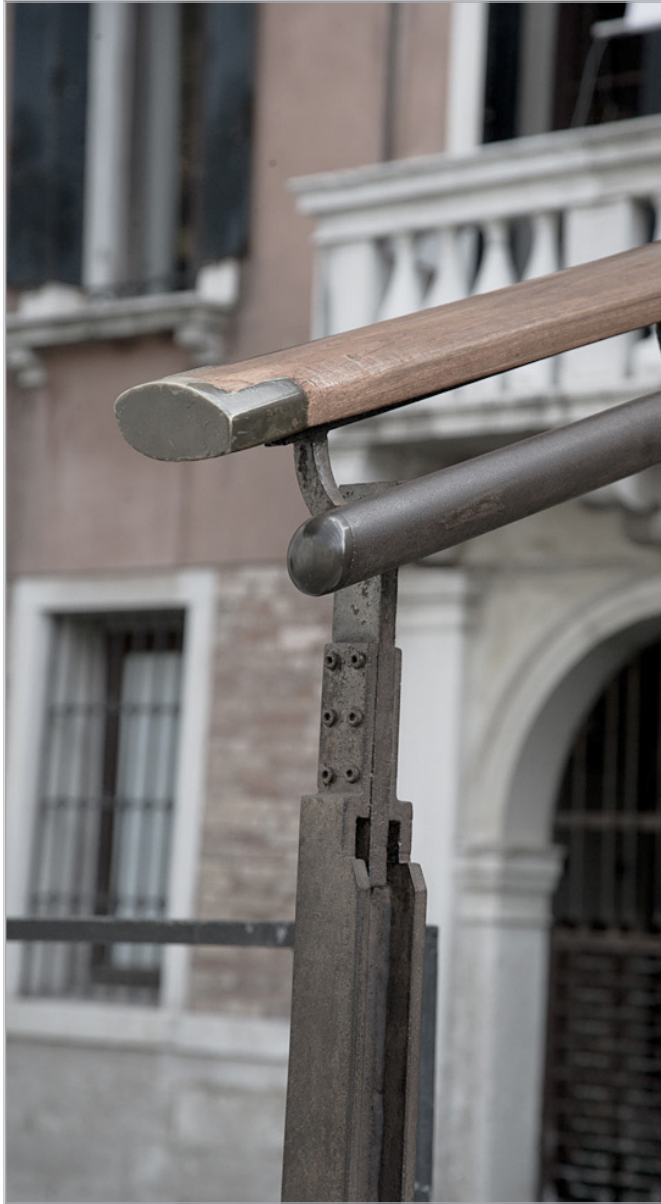
Detail of railing, Querini Stampalia bridge, by Carlo Scarpa
