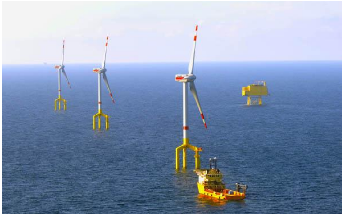
Figure 1 - ABB DolWin Installation, using HVDC connection
