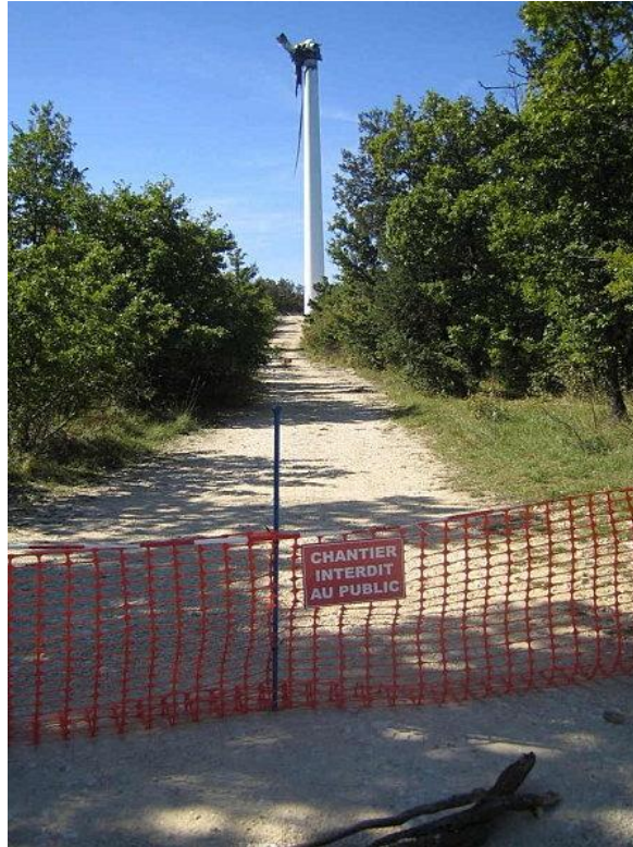
Figure 5: One of the wind turbines which caught fire (Vents Libres sur Nos Collines 2010)
