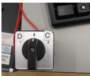
(a) Manual switch for BMS system.
