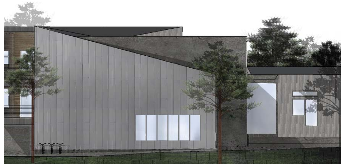
III. 6.5.2 Vertically mounted zinc panels
