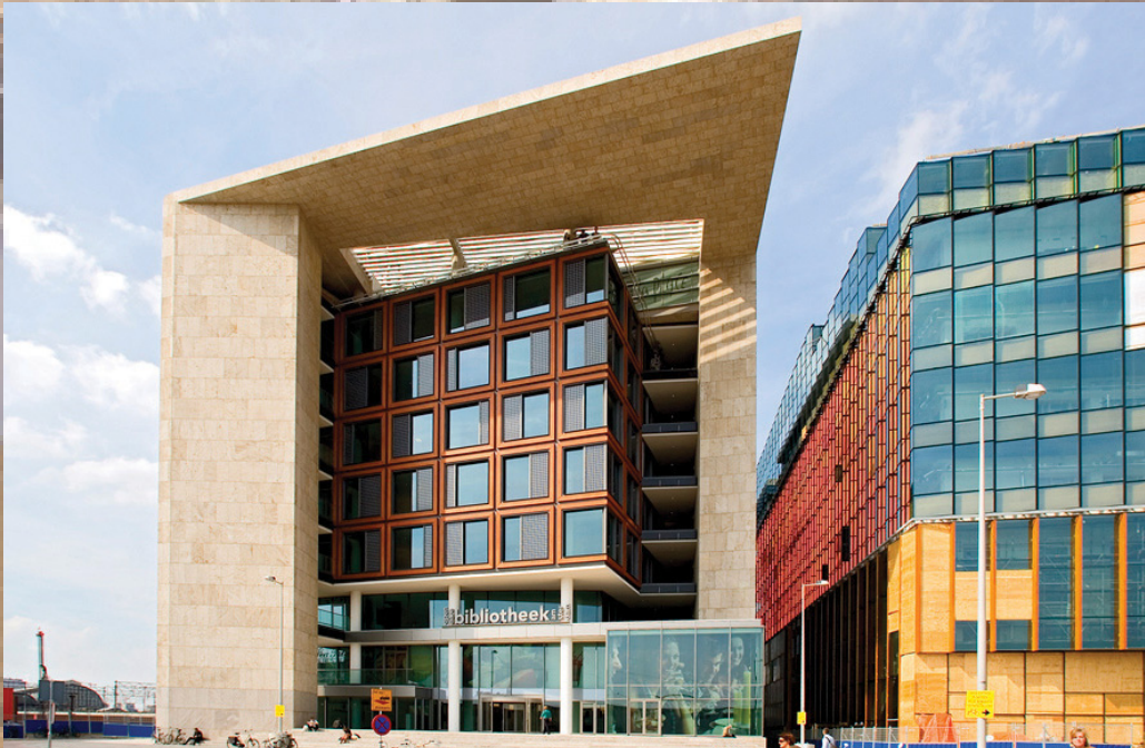
ill. 95 Exterior entrance
