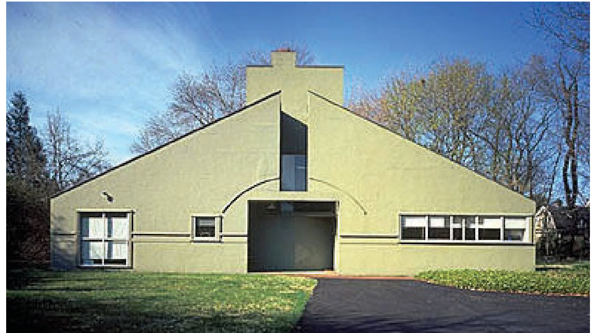
ill. 66 Vanna Venturi House 1962.
