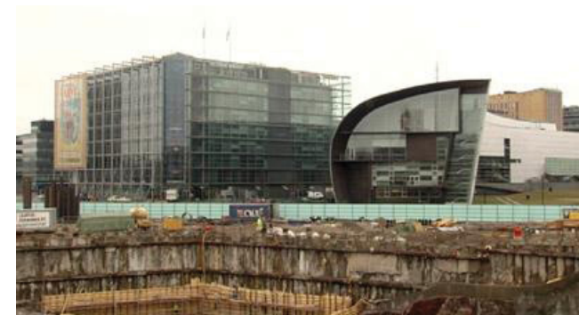
ill. 8 Museum Kiasma and new opera in construction
