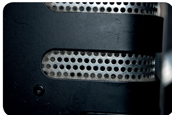
Fig. 50: Dust stored up at the air pocket
