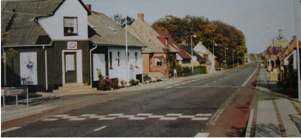
Figure 4.5: Elevated surface at an arterial road in Ullits, Denmark (Rosbach et al. 1996)
