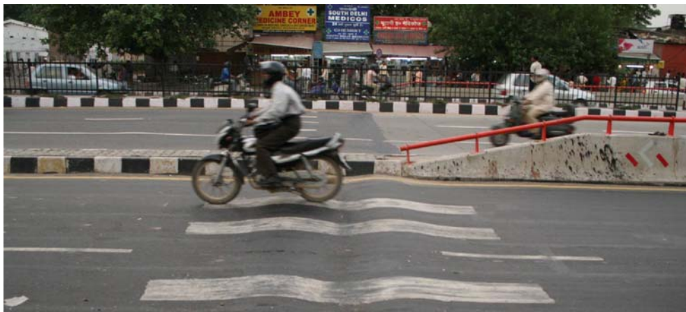
Figure 3.10: A double bump. The driver is without contact with the seat. The only vehicle type that was observed crossing the bump without slowing down the speed was a heavy four-wheel-drive vehicle with soft suspension. The combination of high speed, soft suspension and heavy weight resulted in little influence from the bump.
