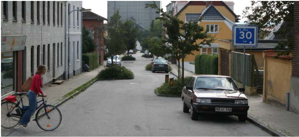
Figure 4.6: Staggering at a local road in Aalborg, Denmark. Only one vehicle can pass through at a time and this type is thus not suitable for arterial roads.
