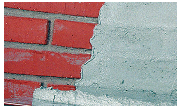
ill. 014 - Muret facade
