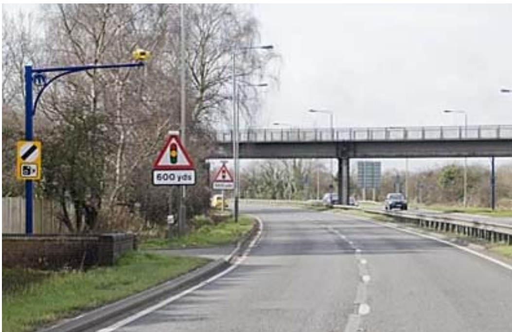
figur A.23: A52 Radcliffe Road (Nottinghamshire Safety Camera Partnership, 2011a)
