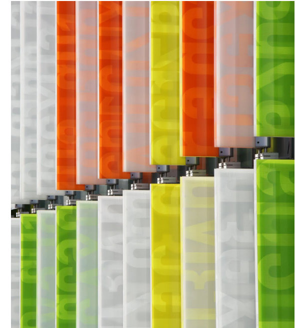
III 344. Coloured solar shading vertical blinds from Ørestads Gymnasiet.
