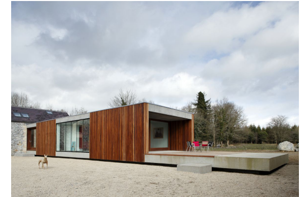
Ill 350. Wood and concrete combination.
