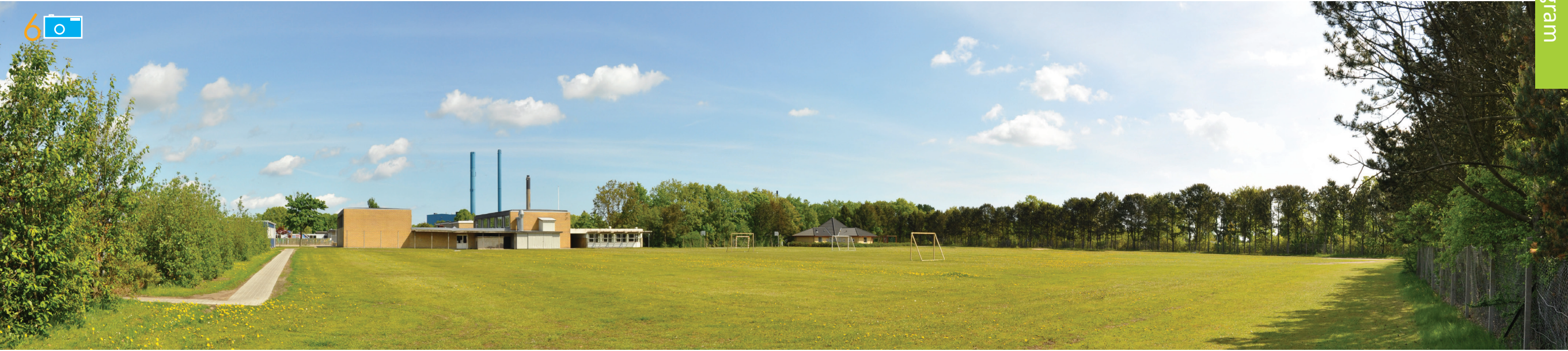
Ill 237. 90° panorama from south west corner of site. the buildings next to the field can be demolished if needed.
