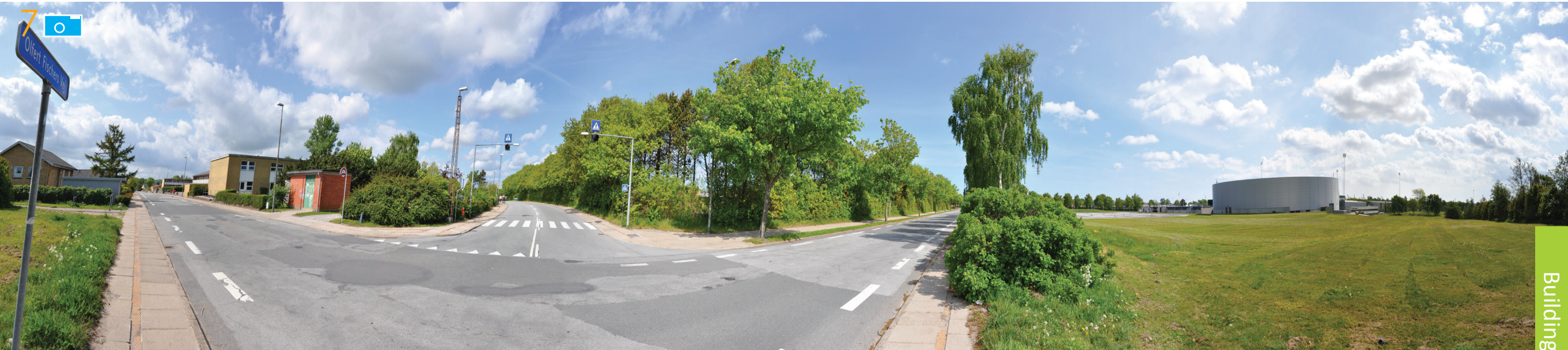
Ill 238. 270° panorama of intersection between Olfert Fischers Vej and Suensonsvej at the south west corner. of the site
