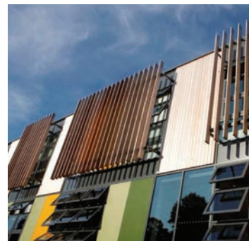
III. 4.43 Vertical louvers 100mm
