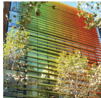
III. 4.41 Horizontal louvers 100mm
