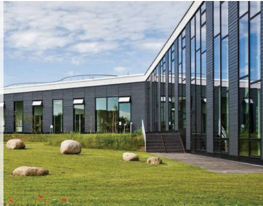
Ill. xx Courtyard of the day care centre
