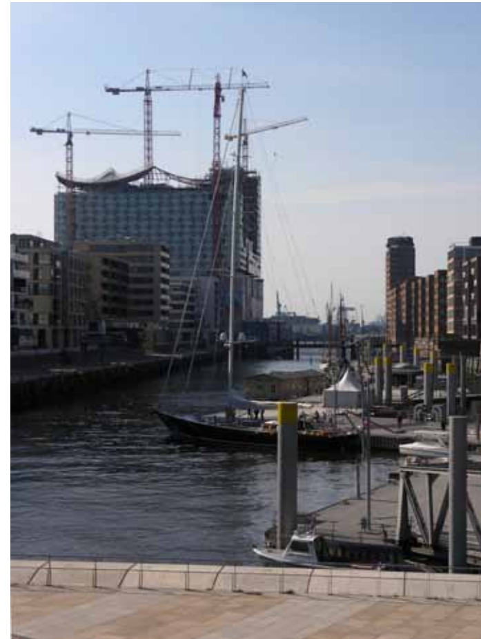
View from Magellanterrassen in Hafencity to Elbphilharmonie
