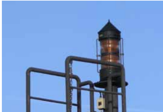
The fresnel lenses of beacons are well visible
