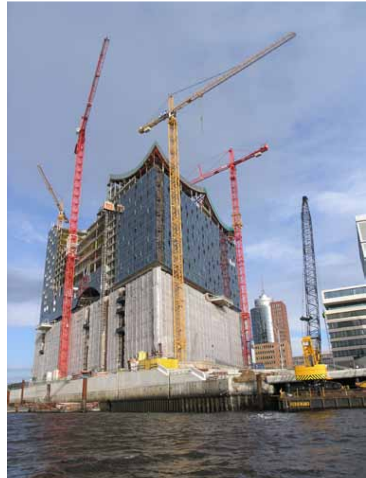
The roof of the Elbphilharmonie showing abstracted waves.
