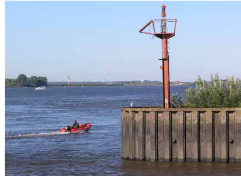
Elbe with lighthouse and beacon in Wedel neighbouring Hamburg to the west
