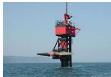
Figure2.8: Real example of tidal current energy converter: Seaflow, Devon, U.K. picture's source Ocean Energy System "OCEAN ENERGY OPPORTUNITY, PRESENT STATUS AND CHALLENGES"
