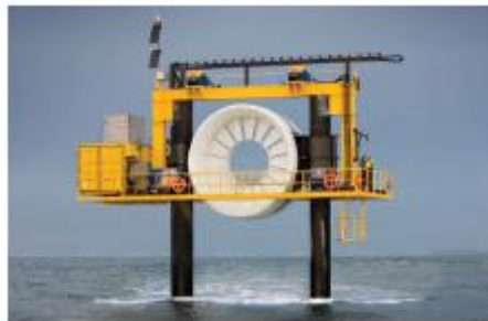
Figure2.10: Real example of tidal current energy converter: Open-Centre Turbine, Scotland picture's source Ocean Energy System "OCEAN ENERGY OPPORTUNITY, PRESENT STATUS AND CHALLENGES"
