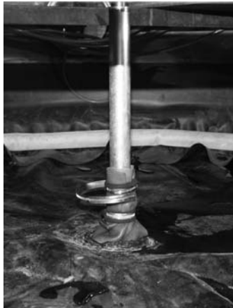
Figure A.7: The pile led through the sealing in the membrane and sealed with two hose clips.
