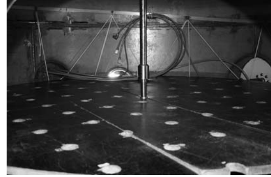
Figure 11: The pile fixed by the hydraulic piston.
