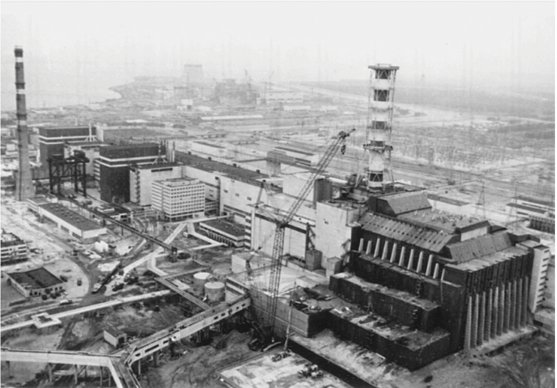
Building of the sarcophagus encapsulation reactor 4.
