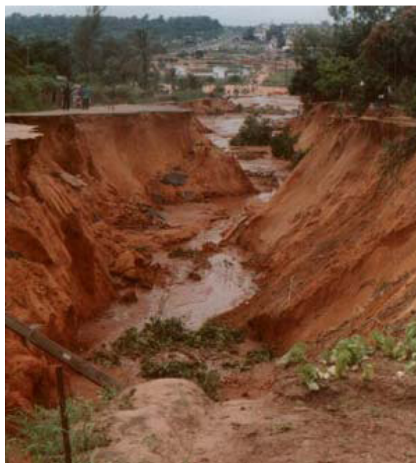
Fig. 4.5 Example of a V-shaped erosion trench
