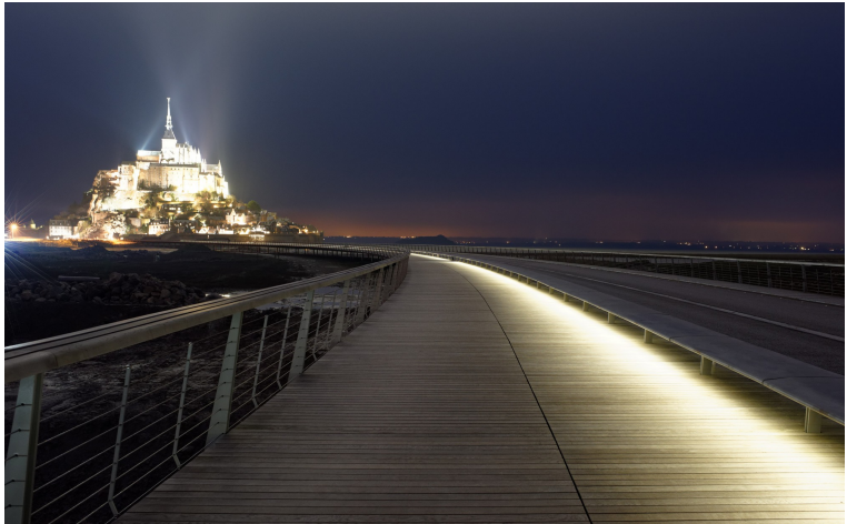
Illustration 24: The Jetty to Mont Saint-Michel. The lighting is embedded into the divider between the pedestrian area and the road. (Photo by: David Boureau)
