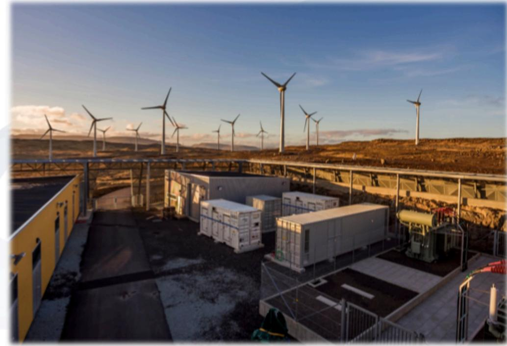
Fig. 19 LEMS battery system at Húsahagi Windmill Park in Tórshavn (SEV 2017)
