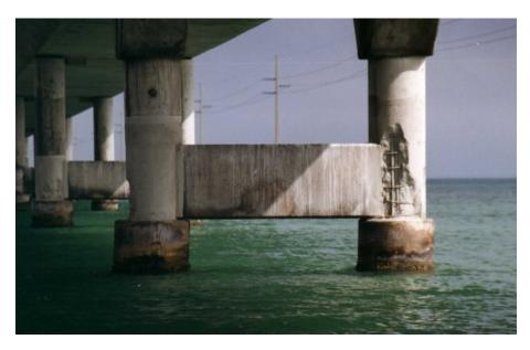
Figure 2.1: Damages in a bridge due to corrosion [13].
