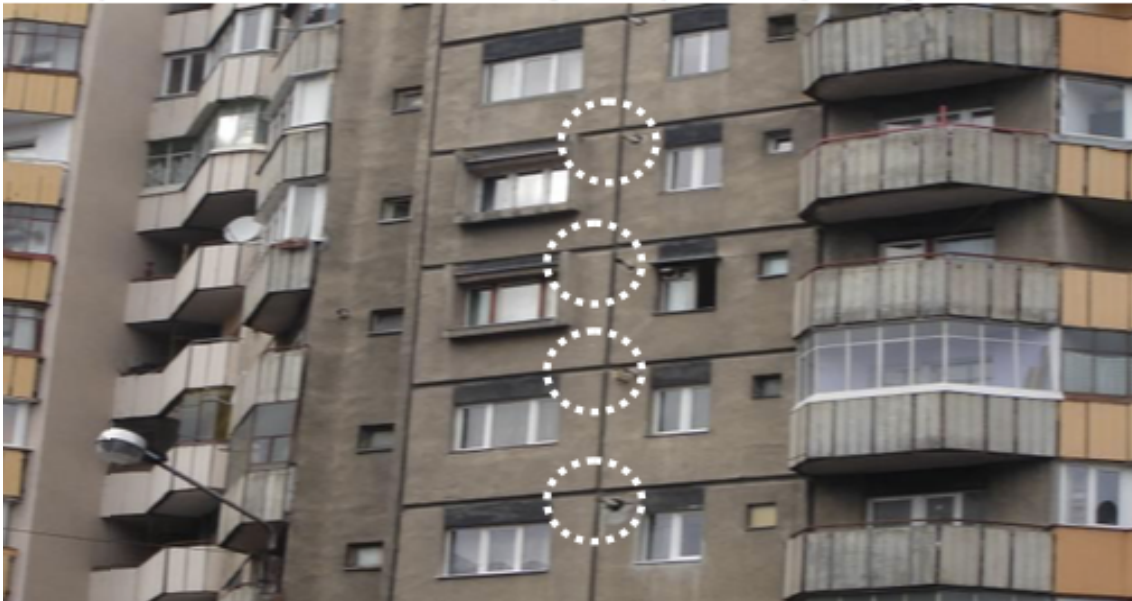
Figure 4.3: Chimneys from individual micro-heating units, protruding through outer walls (Ministry of Regional Development and Public Administration , 2013)
