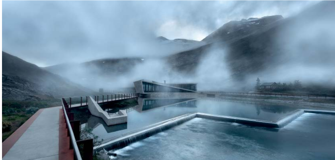
Ill. 13: Trollstigen main building with regulated cascades in the front.
