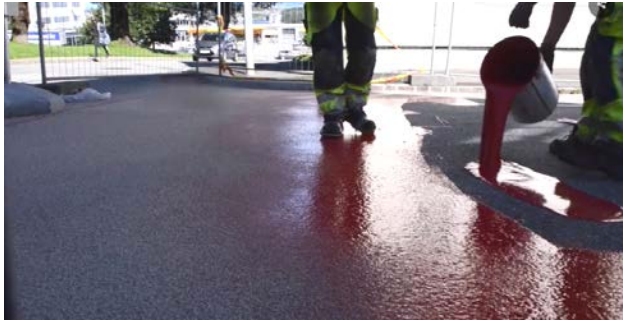
Figure 8: Construction of Bicycle Priority Street, Stavanger (Stavanger Aftenblad, 2016)
