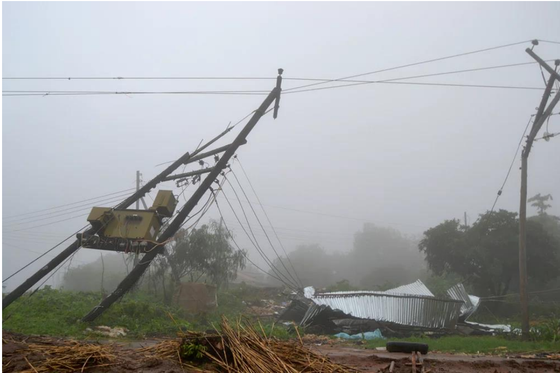
Figure 3 Destroyed infrastructures by the floods
