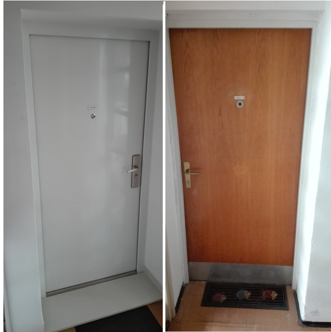
Figure 2.3: An example of old and new entrance doors of apartments ( Photo from field visits )
