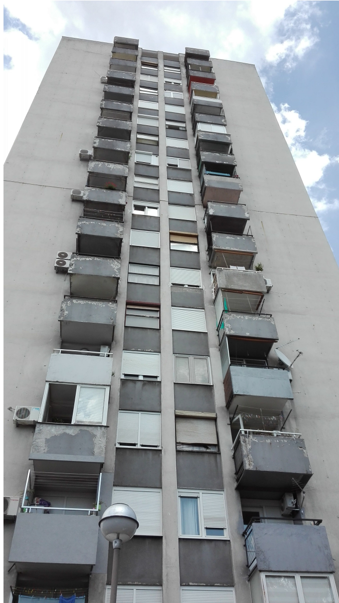
Figure 4.5: External walls between windows
