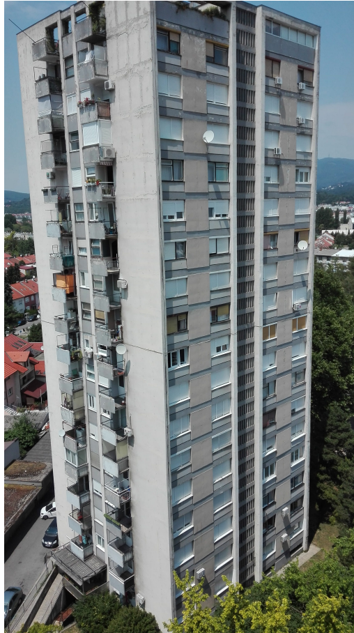
Figure 2.4: The selected residential building in Zagreb ( Photo from field visits )
