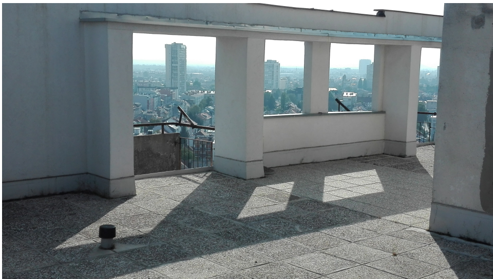
Figure 4.7: A part of the terrace with a poor insulation ( U = 2 \text{ W/m}^2\text{K} )
