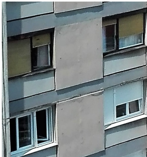
Figure 2.2: An example of old and new windows ( Photo from field visits )
