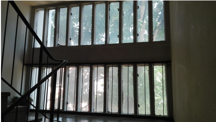
Figure 4.8: Staircase windows at the first floor
