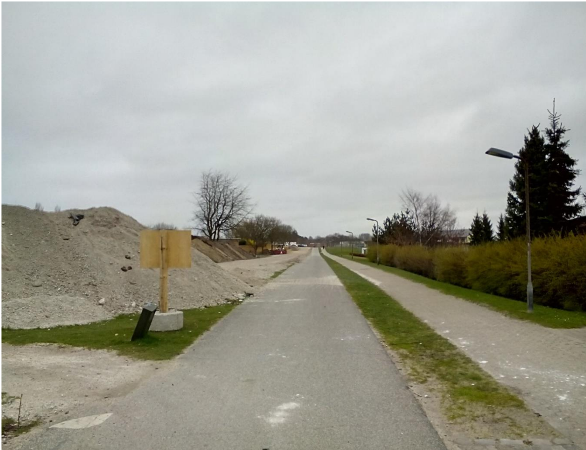
Image 13: “New Aalborg East” under construction together with Astrupstien link
