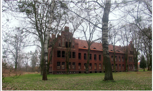
Owinska Mental home, where some of the first victims at Fort VII came from, now derelict and falling to pieces (own photo)
