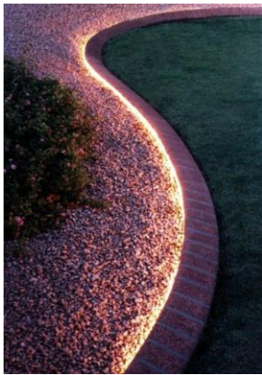
Figure 26: Ground recessed LED strips
