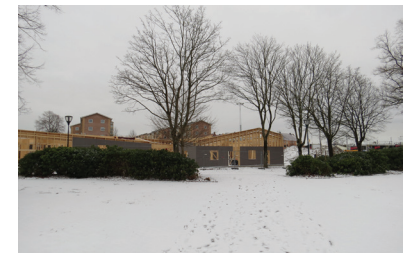
III.22: 8. The new building under construction
