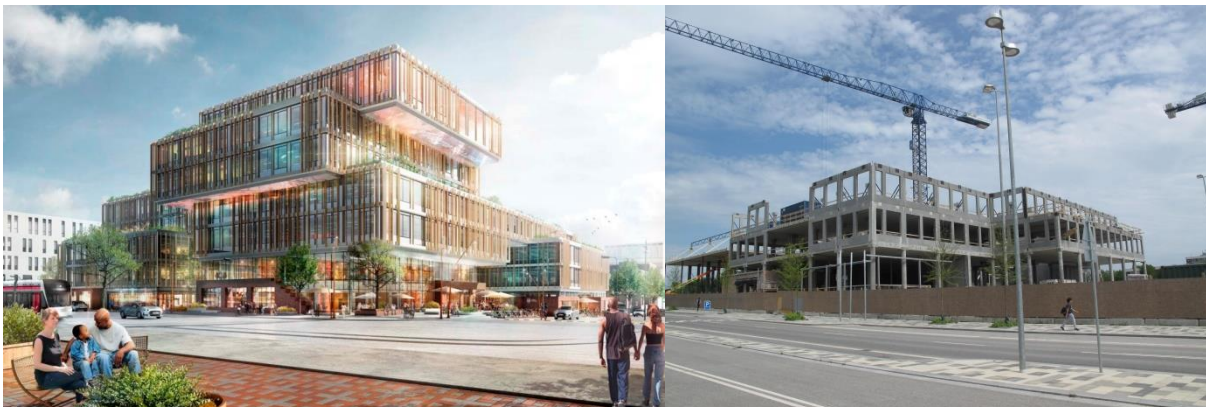
Picture 11 and 12: The Meet Aarhus project. Visualization (OpsGellerup n.d. a) and under construction.
