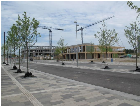
Picture 7: Karen Blixens Boulevard, Gazellefarmen and Meet Aarhus under construction.
