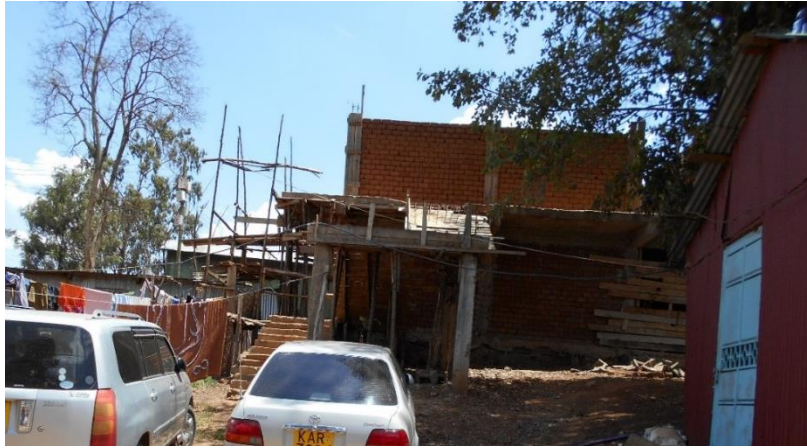
Figure 22: Stalled 'Waiguru toilets'. This was a WATSAN initiative throughout the Kibera settlement started by the Ministry of Devolution ca. 2014. It involved building of roads, sewers and ablution blocks. Political discontent and rumours of corruption clouded the project. (Source: Author)
