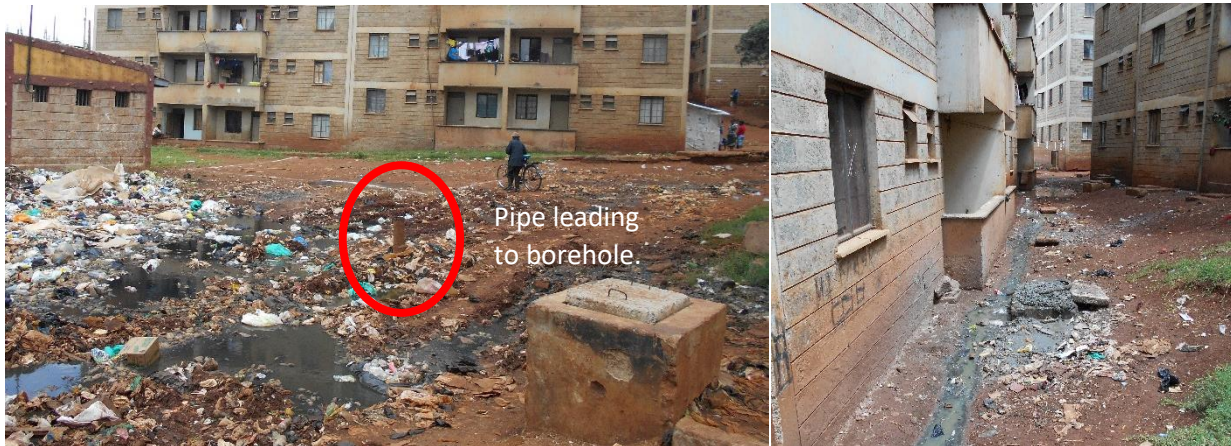
Figure 15: (a) The abandoned borehole that was to provide water to the decanting site. The area has now become a solid waste dumping site. (b) Overflowing sewer lines. Occasionally, the residents would clear it up themselves. (Source: Author)
