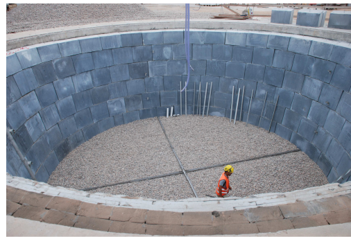
Figure 1.9: The 100 MWh CSP pilot plant in Ait Baha, Morocco (Zanganeh, 2014).
