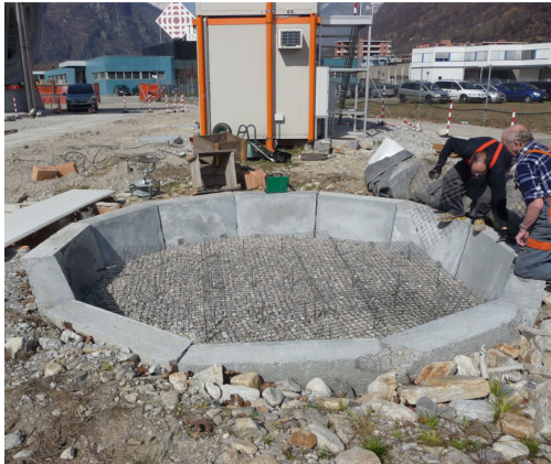
Figure 1.8: The 6.5 MWh pilot plant at Biasca Research Facility, Switzerland (Zanganeh, 2014).
