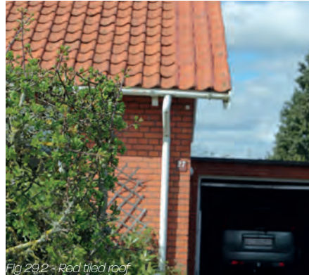
Fig 29.2 - Red tiled roof
