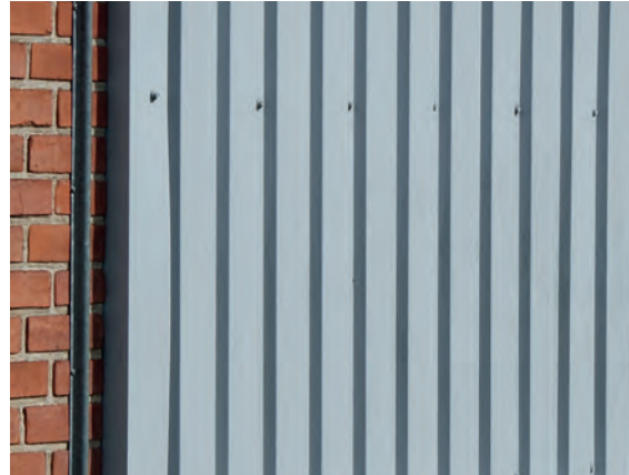
Fig 28.2 - Sinus steel plates
