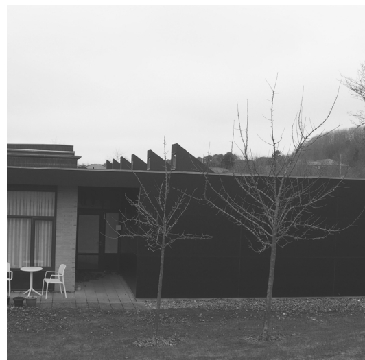
III. 32 On all north oriented residences a south oriented skylight is mounted on the otherwise flat roof.
