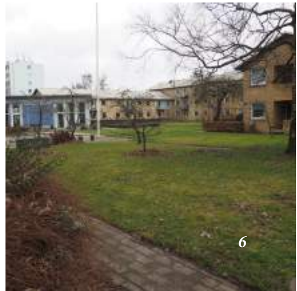
III. 43 Interior courtyard in the existing nursing home.
