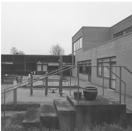
III. 31 The courtyard in the main building is simple means of exercise, for example a staircase with varying inclinations.
