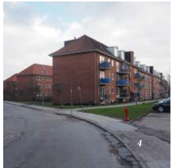
III. 41 Renovated elder housing.
