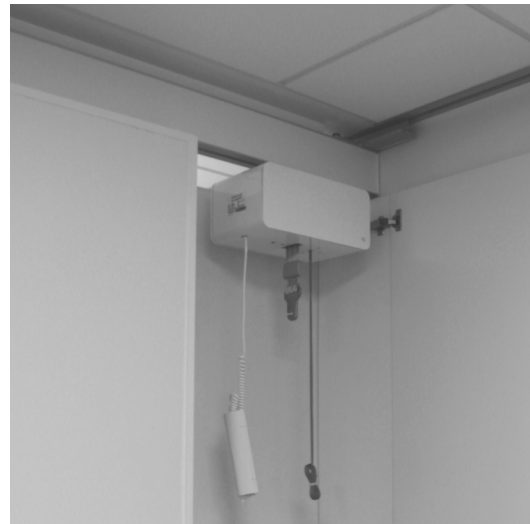
III. 23 The lift is parked in a double sided closet accessible from both the toilet and bedroom.
