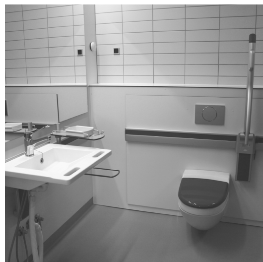
III. 24 All interior in the toilet is installed on flexible mounts for adjustment to the user.
