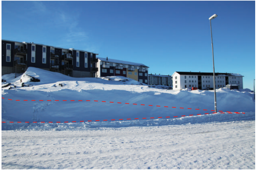
Fig. 19: View from north-east towards the site with the neighboring dwellings
