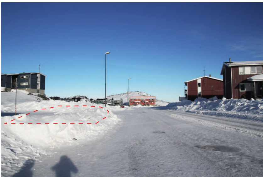
Fig. 15: View from access road towards North with the site on left hand
