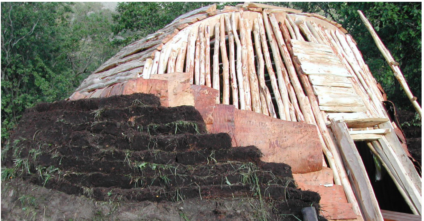
▼ Illustration 18.1. Construction of goahti
