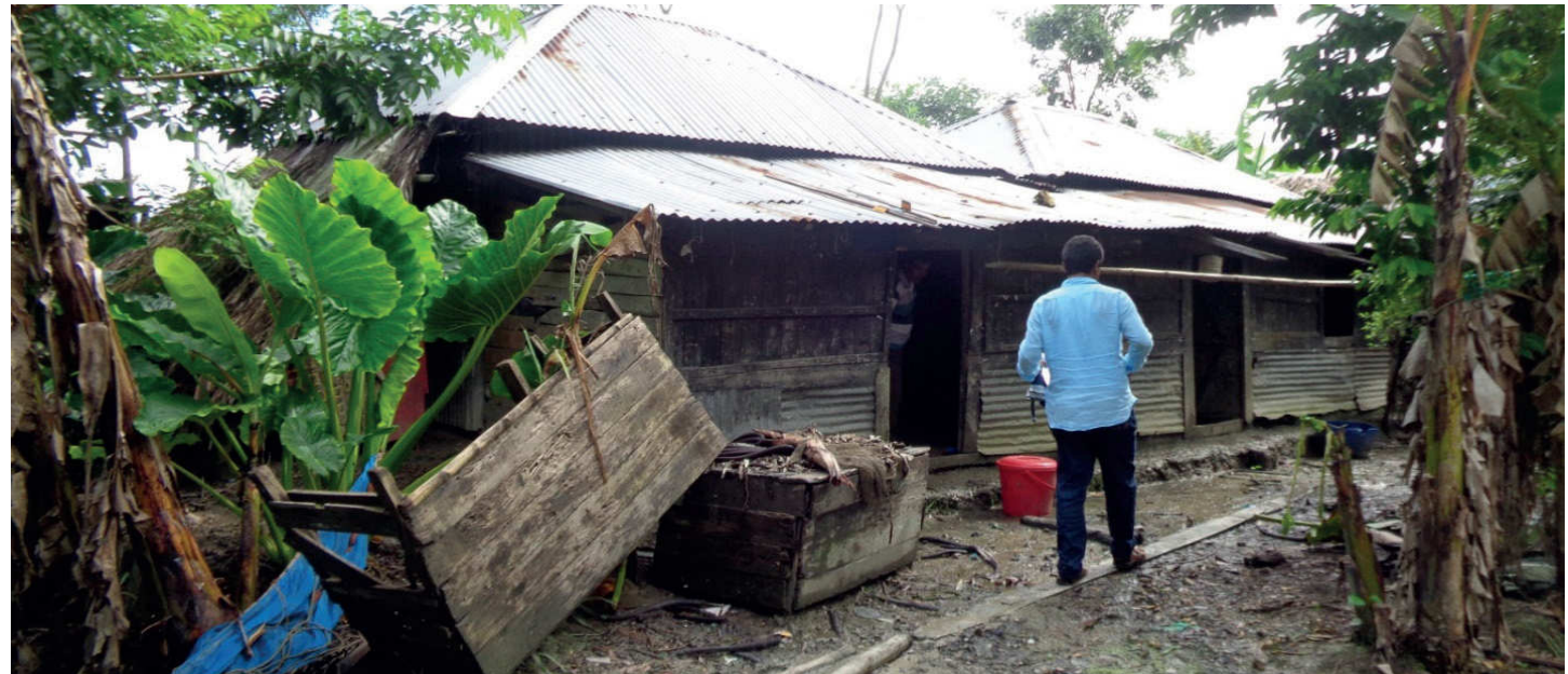
FIG. 36: A HOUSE IN THE COASTAL VILLAGE WITH HIPPED PITCHED ROOF MADE OF CI SHEETS
