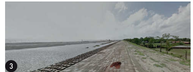
FIG. 11: EMBANKMENT NEAR THE SEASIDE
