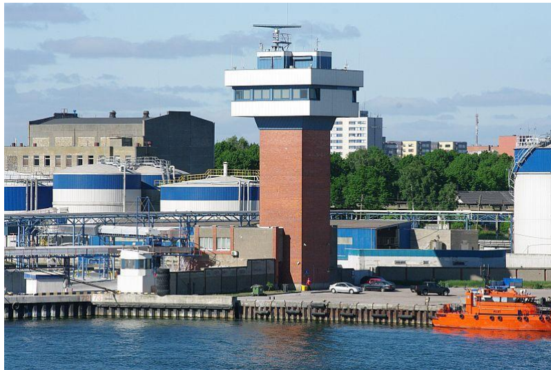
Figure 11. KSSPA's Vessel Traffic Service tower. 21
