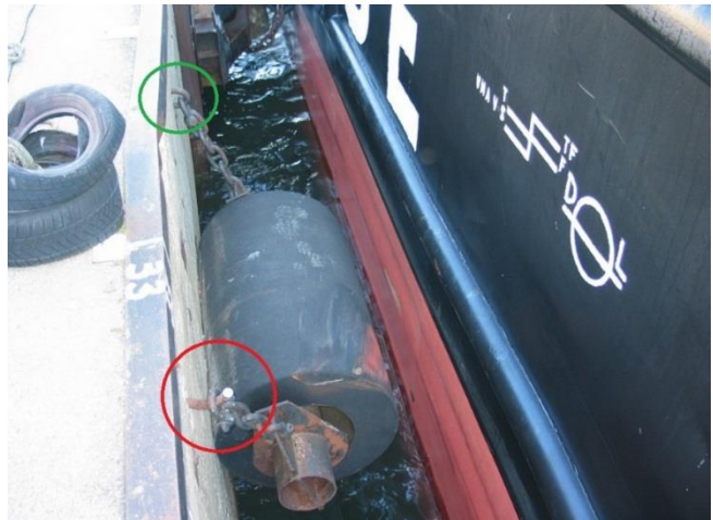
Figure 13. Metal loop broken on which rubber fender is hanged
