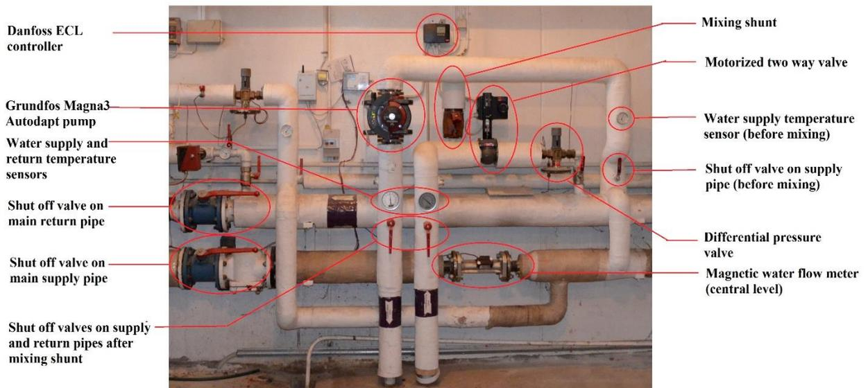
Figure 3.6 District heating connection for the ground floor of the East block
