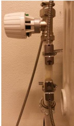
Figure 3.29 Clamp-on flow sensors
