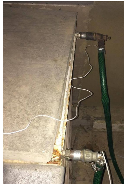
Figure 7.4 – Picture of water pipe connected to radiator
