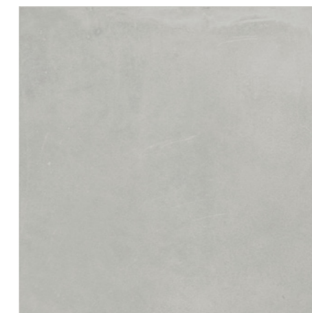
III. 05.14 Polished concrete floors
