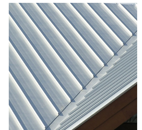
III. 05.13 Zinc roofing
