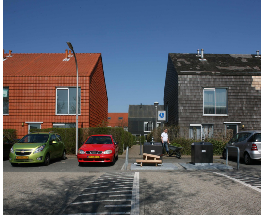
III. 9.2 Heterogenous cladding, Ypenburg ,Rotterdam
