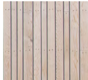
Figure 21, Thermal treated pine on the sheds and community house's facades
