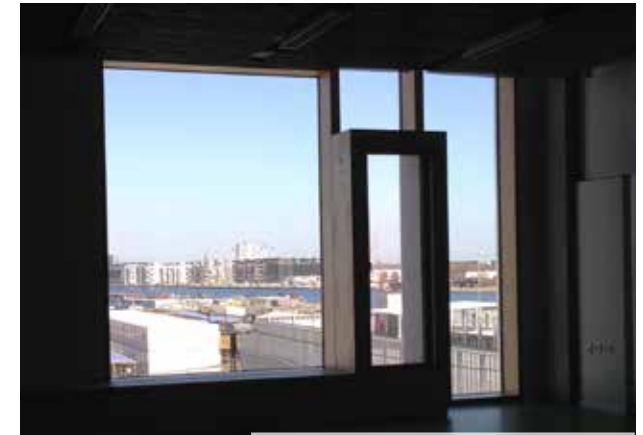
Window in classroom III.26
