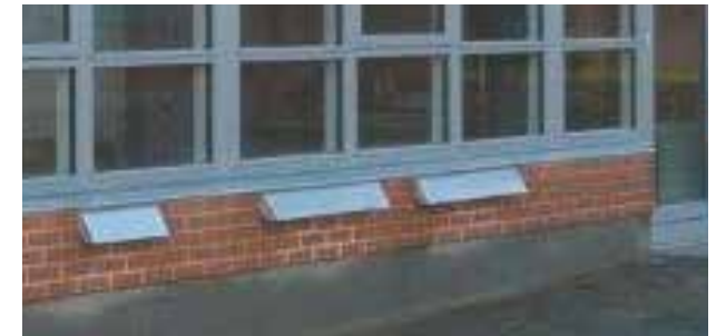
InVentilate placed under window, seen from outside Ill. 49
