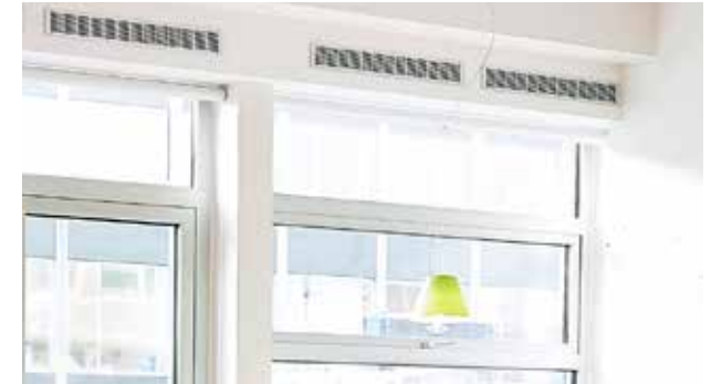
InVentilate placed over window, seen from inside Ill. 48
