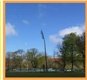
High masts with downward spotlighting, sport courts.
