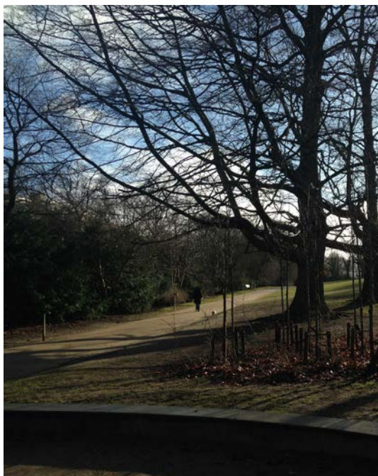
Figure 38. Photo of the bollard luminaires where measurements were taken
