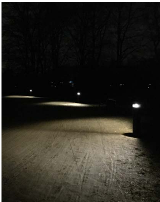
Figure 14. Photo of the bollard luminaires where measurements were taken
